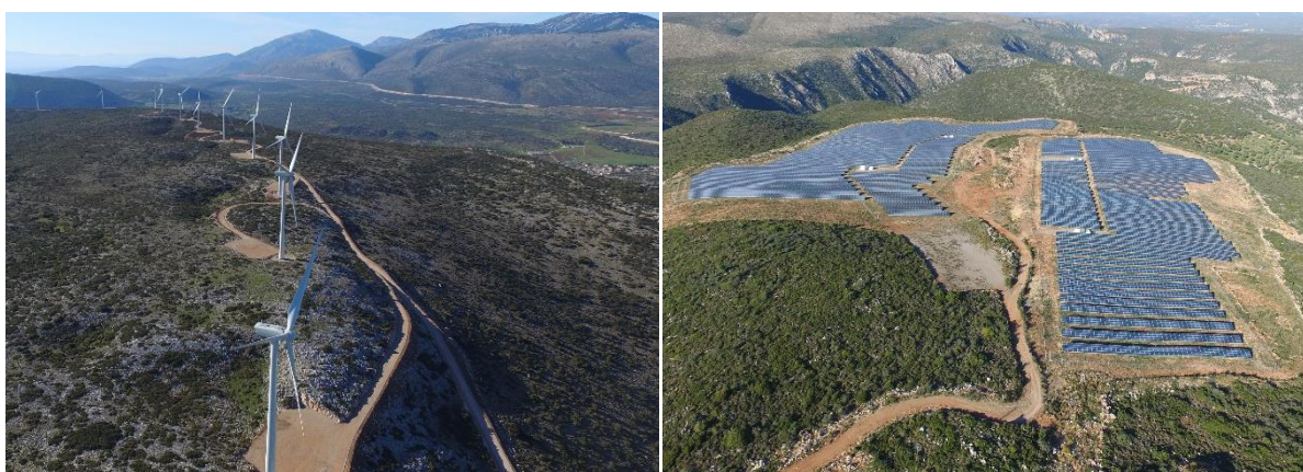
Maristi (42 MW) and Paleochora (9 MW) power plants in Greece (© Total Eren)
